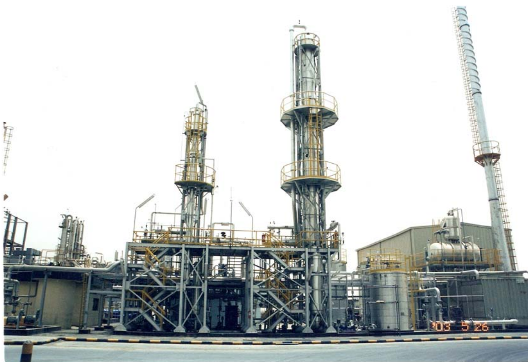
SFCCL (Chemanol), Excess Water plant
